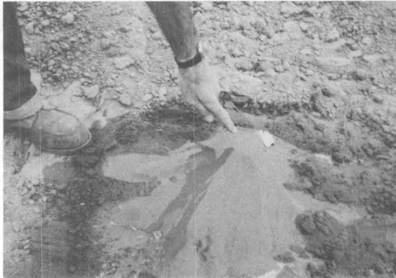
Figure 26. Sand boil formed from dissipation of pore water pressure in silty sand.
