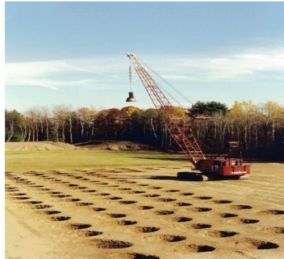
Figure 1 – Typical Dynamic Compaction Grid Pattern
