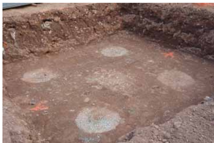
Figure 3: Typical stone column layout and footing location.
