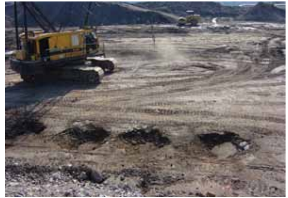
Figure 4: General photograph of dynamic compaction.
