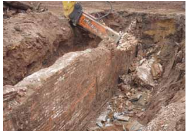
Figure 1: Typical foundation remnants on an urban site.
