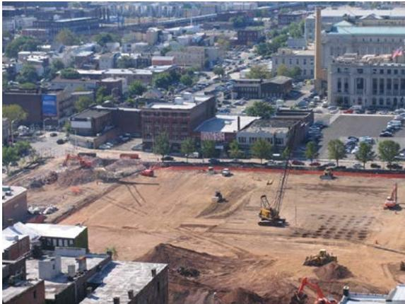
*Figure 10 – Dynamic Compaction Production*
